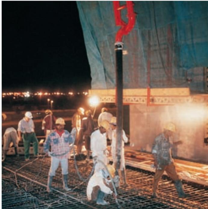
Such night-time pours as seen here are typical in the UAE and many other countries where the daytime temperatures are very high. Working at night is not only cooler for the personnel but assists in reducing the temperature of the concrete placed. Night-time pours are also a useful means of avoiding the day-time traffic jams where concrete is delivered from off-site batching plants.
