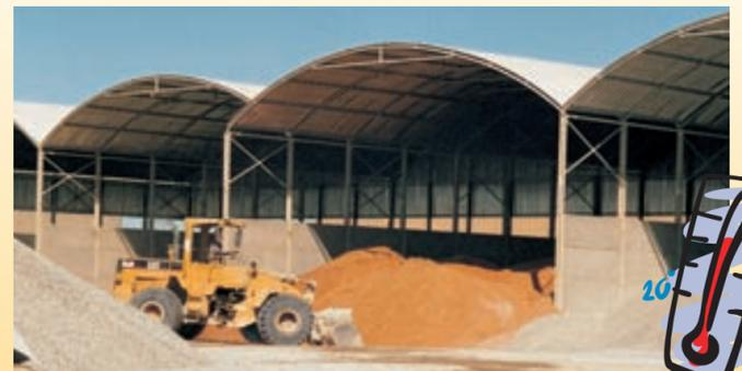
For this project the aggregate storage area was covered with sun shades and cooled water used to make the concrete, in order to stay below the maximum allowed concrete placing temperature. In Dubai and other countries with high temperatures and high sunshine ratings, when a relatively low concrete
