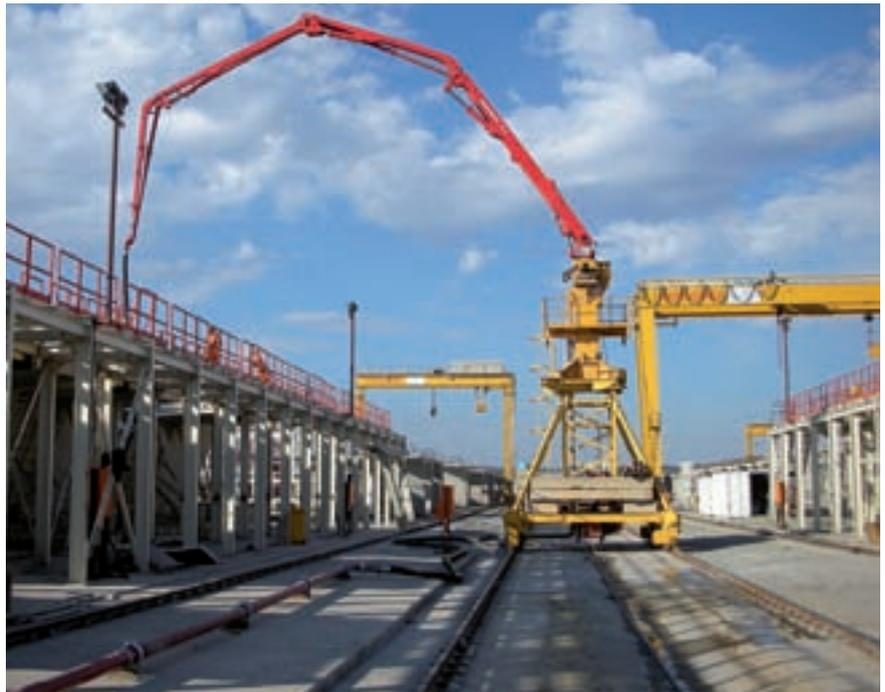
The Putzmeister MX 24 stationary boom on rails spreads the concrete in the moulds of the prefabricated elements
